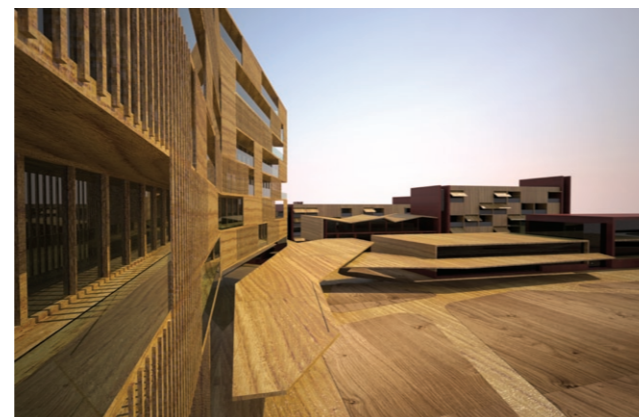
Port Hedland, WA - medium density, mixed-use development
